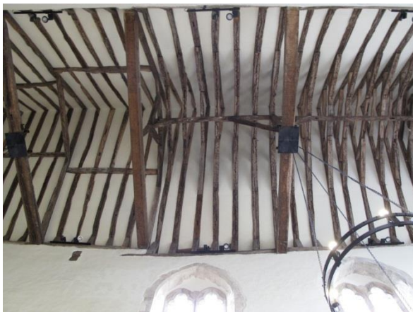
The interior roof beams and braces
